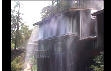
Figure 2-8. FireMaster System in action [5].
