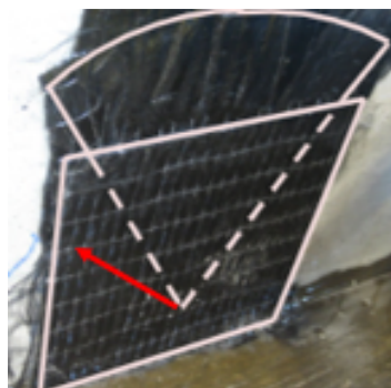
Figure 3.4 – FRP Splay Anchor Under a Wall [18]
