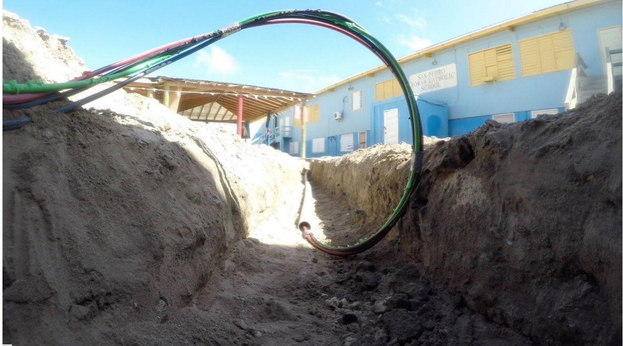
Figure 1: Crew 1 (mine) was tasked with conduit runs and wire pulling.
