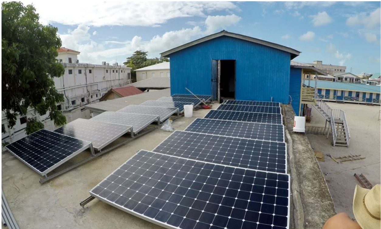
Figure 2: Crew 2 mounted the panels.
