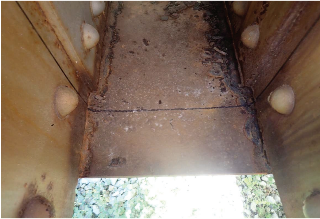
Photo 21: Bottom batten plate at Cross Section 3
