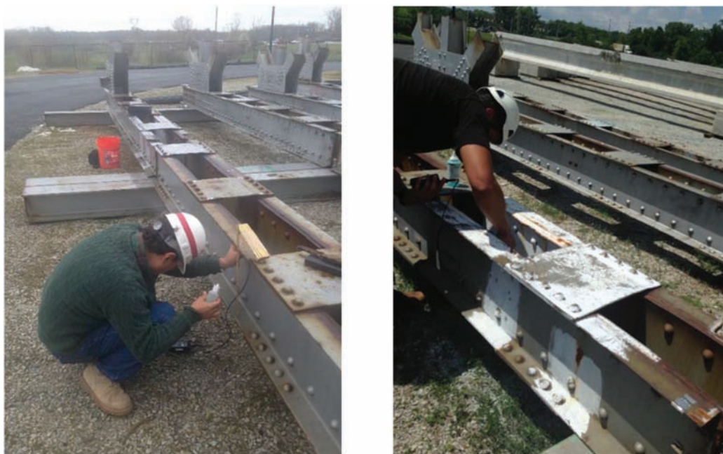
Figure 7.2 Two inspectors taking thickness measurements of the truss chord.
