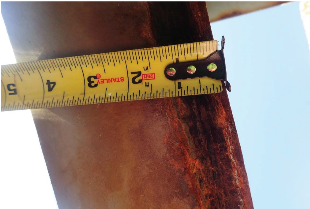
Photo 12: Channel A at Cross Section 1 (bottom)
