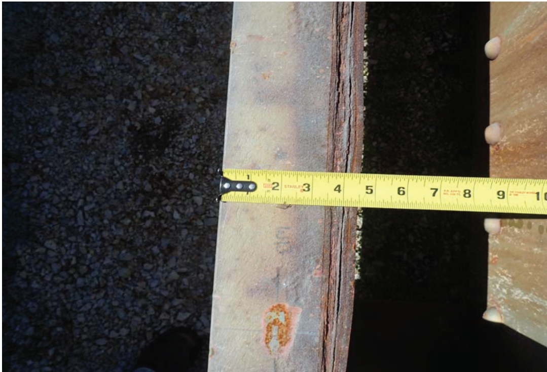
Photo 14: Channel A at Cross Section 2 (top)
