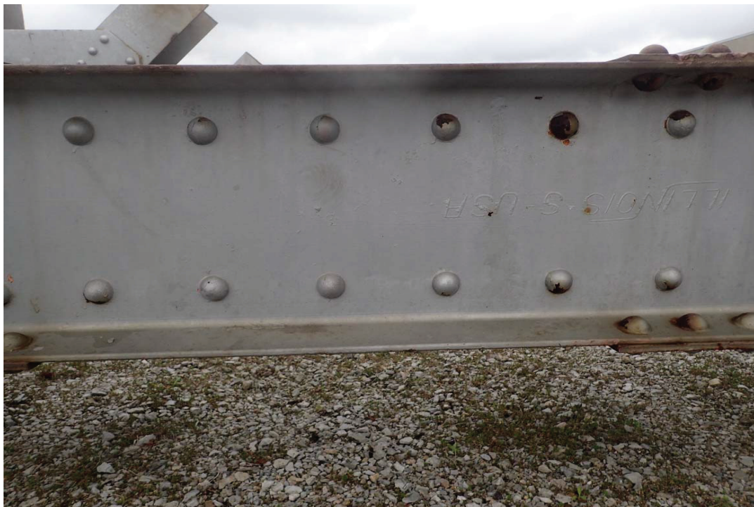
Photo 4: General condition of exterior face of channels (Channel A)
