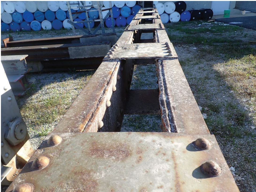
Figure 2. Truss chord plan view (looking from joint L4 toward joint L2)
