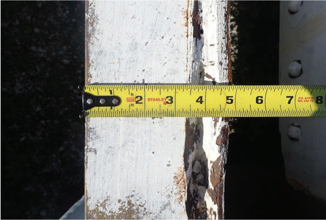
Photo 9: Channel A at Cross Section 1 (top)
