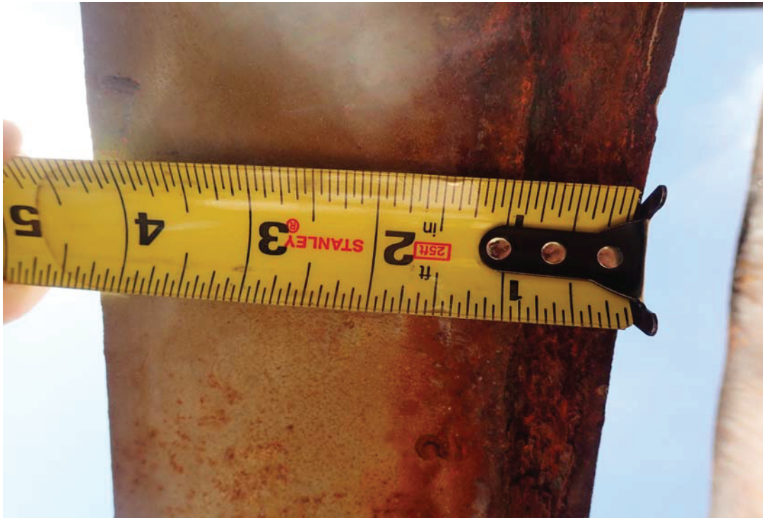
Photo 16: Channel A at Cross Section 2 (bottom)
