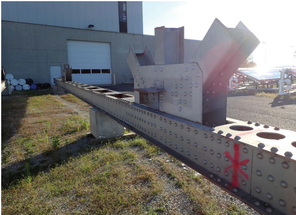
Photo 2: Bottom Truss Chord (Member L2-L4)
