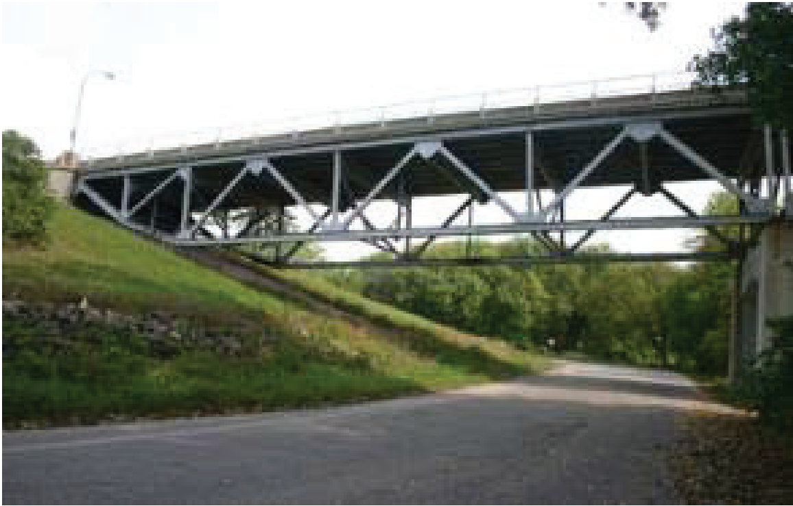
Photo 1: Elevation View of Approach Span 16
