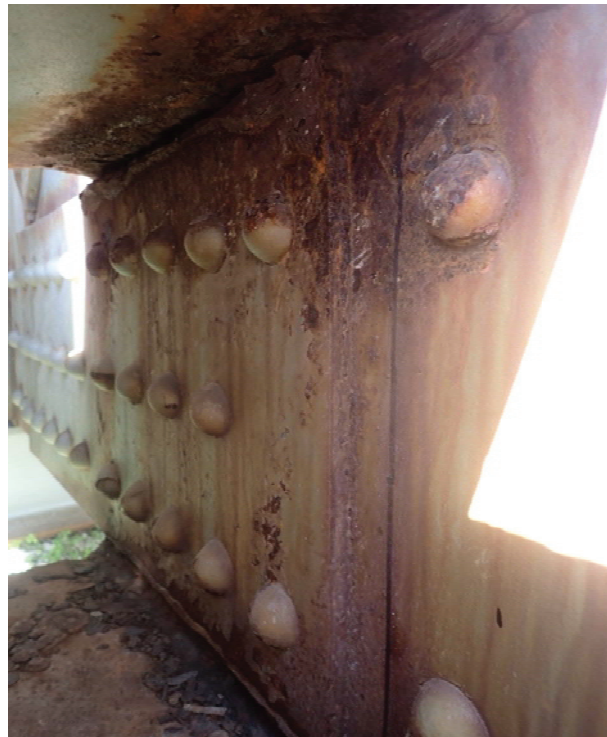
Photo 22: Web and splice plates on Channel B at Cross Section 3
