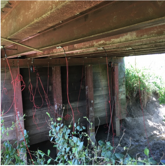
Fig. 14. Transducers attached to girders
