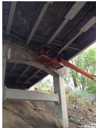
Fig. 3. Boom truck operating under the bridge
