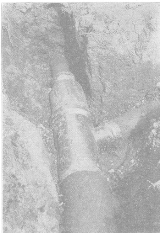
Fig. 8.—A sewer “Y” and a 6"x 4" sewer reducer make a perfect junction of a 4" and a 5" line to a 6" main.
