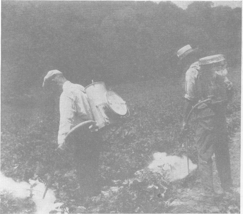
Fig. 9.— Knapsack bellows type of dusters for truck gardens.
