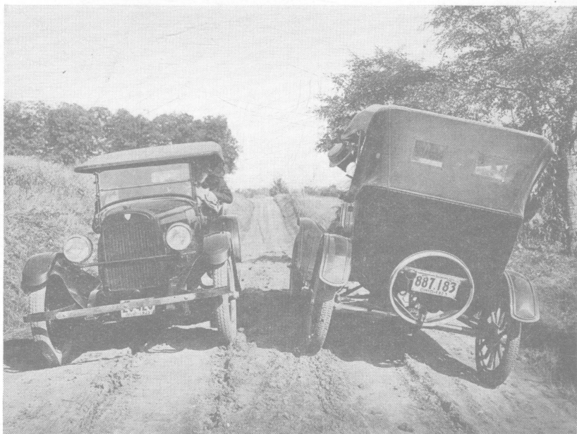
Fig. 2.—Wrong method of earth-road grading. Crown is roof-shaped and too narrow. It is dangerous when surface is slippery
