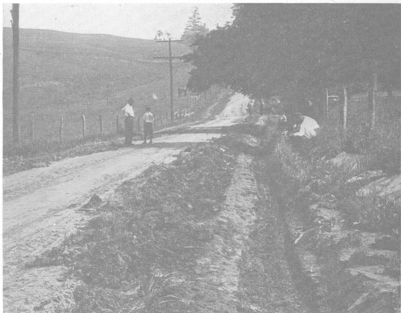
Fig. 7.—Ditch is being deepened in second round. The loose earth is moved over the top of sods
