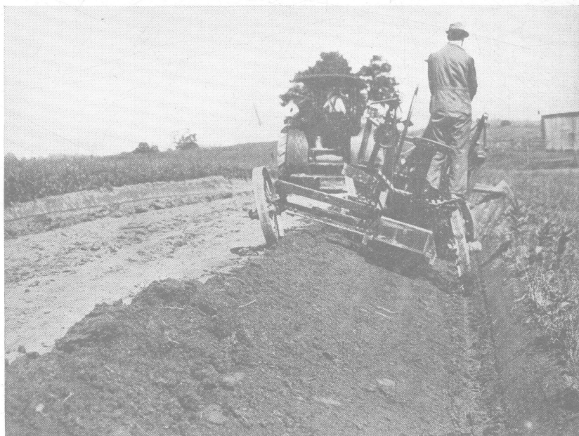
Fig. 11.—Giving the finishing touch to the side ditch
