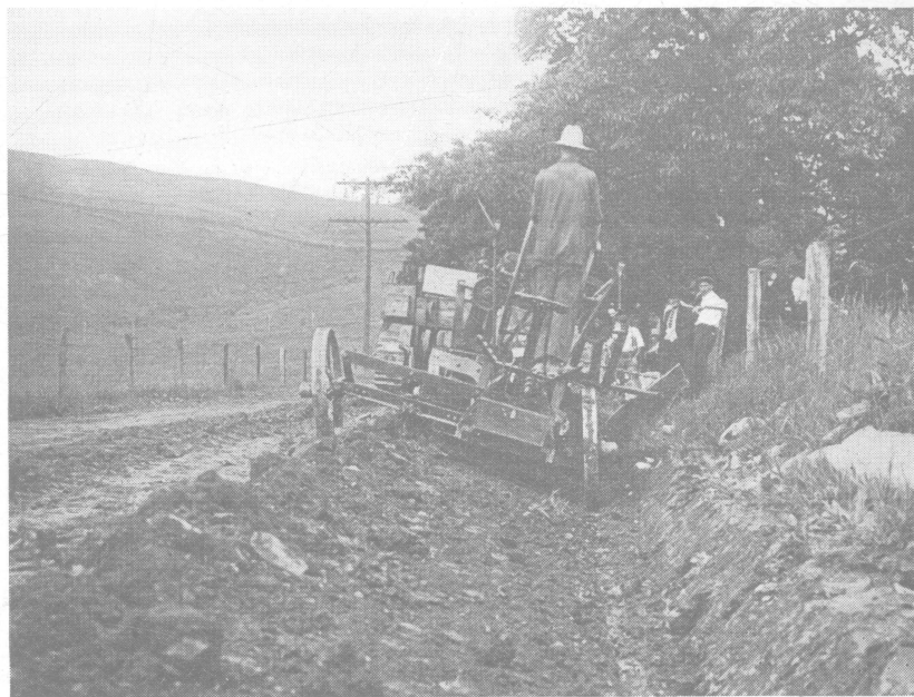
Fig. 8.—Back sloper attached in third-round operation; first step in shaping side ditch
