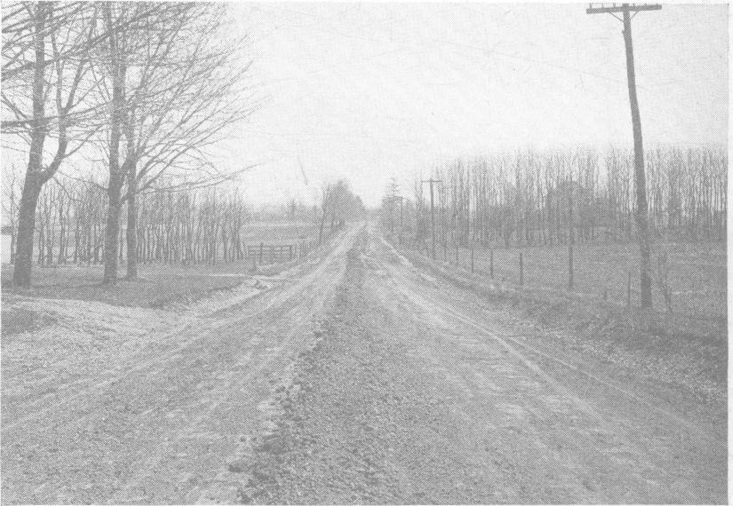
Fig. 16.—Graded road after one year's service with consistent maintenance
