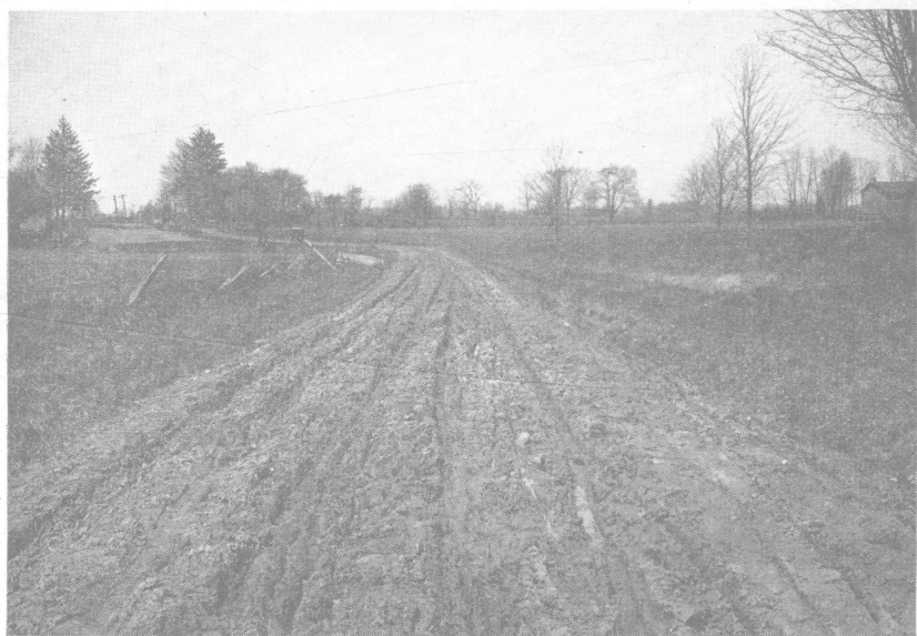
Fig. 18.—Road upon which both grading and maintenance have been neglected
