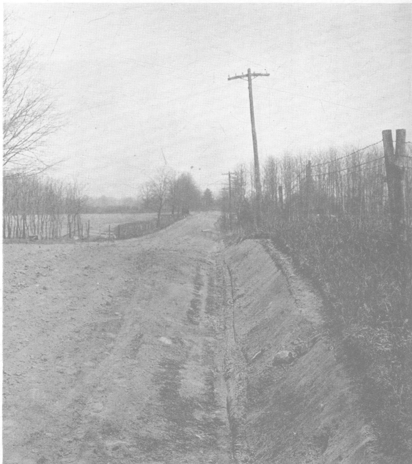
Fig. 14.—Ideal side ditch construction of graded road
