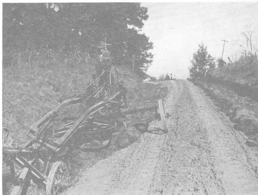
Fig. 6.—Another view of the first round, showing how sods are cut and properly placed
