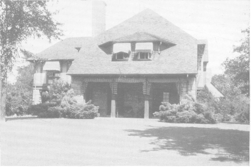
Fig. 2.—A house that is a home! These simple, yet very effective corner plantings, are composed of two Pfitzer and a spiny Greek Juniper.
