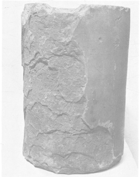
Clay tile damaged by frost.
