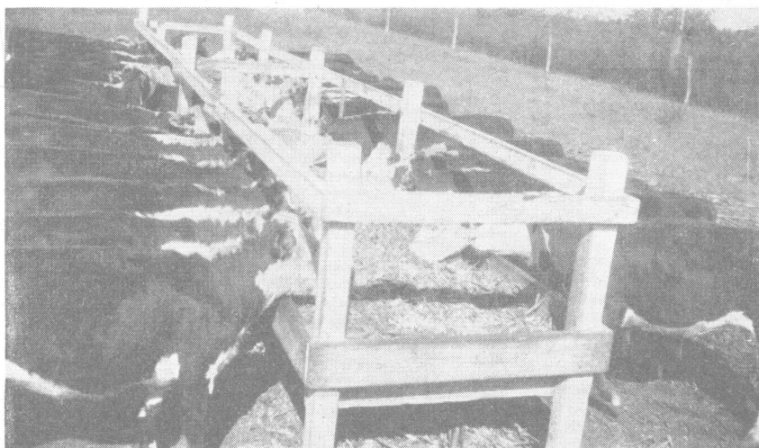
Fig. 13.—Feed bunks must be made of heavy timbers and solidly put together in order to stand up under hard use.
