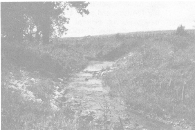
Rip rap and vegetation control erosion in the Dorn drainage project, Madison County.
