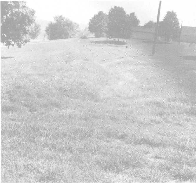
Completed diversion terrace with well established vegetation.
