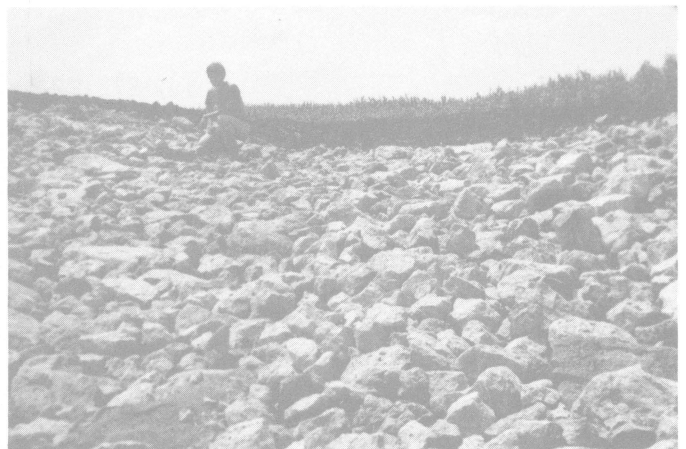
Rip rap chute for erosion control where water runs over ditch bank.
