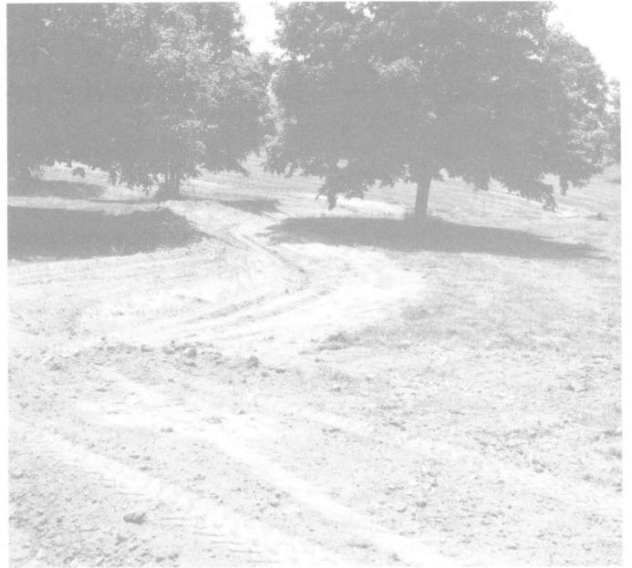
Diversion terrace under construction for erosion control in Noble County.
