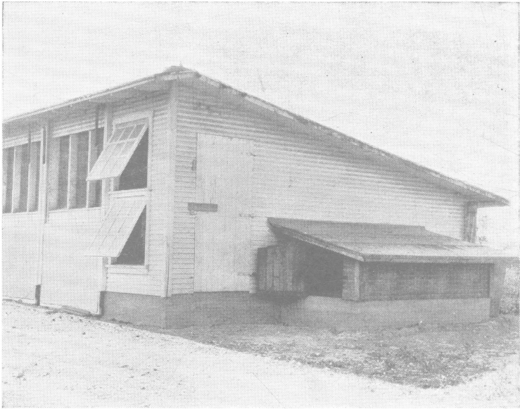
Fig. 10.—A small addition to the house, similar to this, is all that is necessary to house the heating unit for a poultry house. Fig. 9 shows the heating unit.
