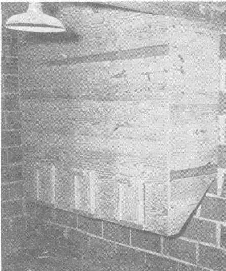
Fig. 18.—Wall feed bins save floor space and prevent feed waste. They can be filled from the outside.
