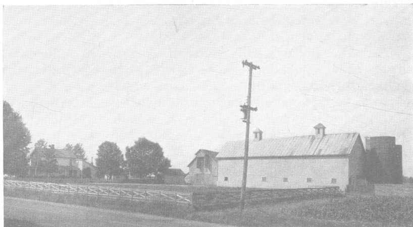
Figure 1.—Home of Leo Coleman, one of the largest users of electricity on the Marysville line. The transformer (box on the pole in the foreground) steps down the voltage from 6600 volts to 110-220 volts.
