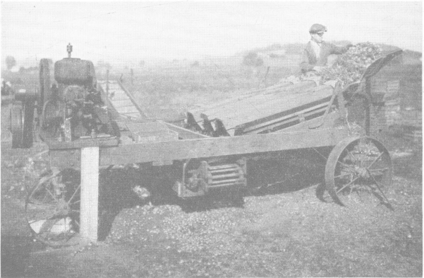
Fig. 10.—Onion toppers afford an economical means of removing the onion tops.
