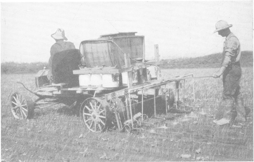
Fig. 22.—Home made onion sprayer suitable for large acreage.
