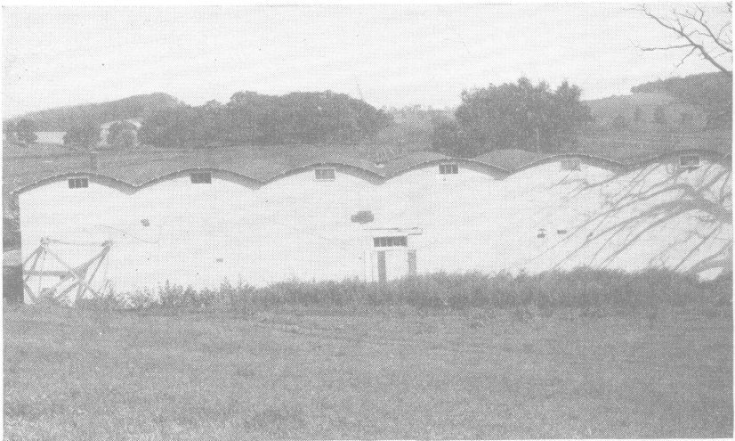
Fig. 15.—An onion storage house. Note windows and ventilators.
