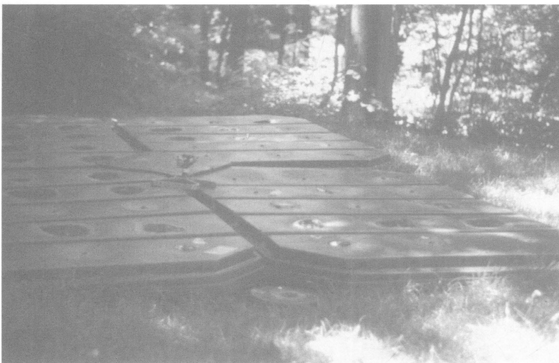
Figure 5. Examples of roofs used for bioreactors in Ann Arundel County, Maryland.
