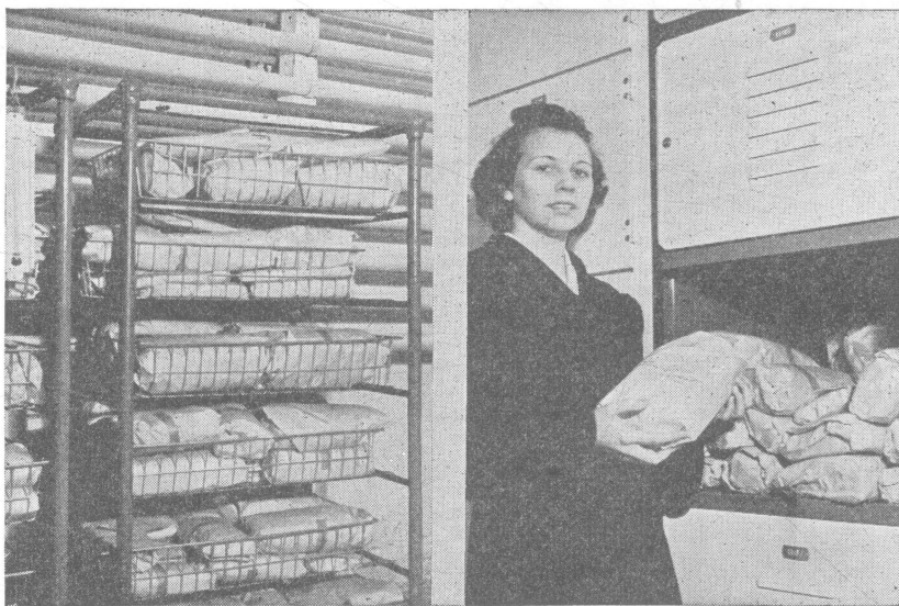
Interior of a commercial freezer locker plant. At the left, trays for packages in the quick freezer. At the right, a patron removing packages from a typical locker.
