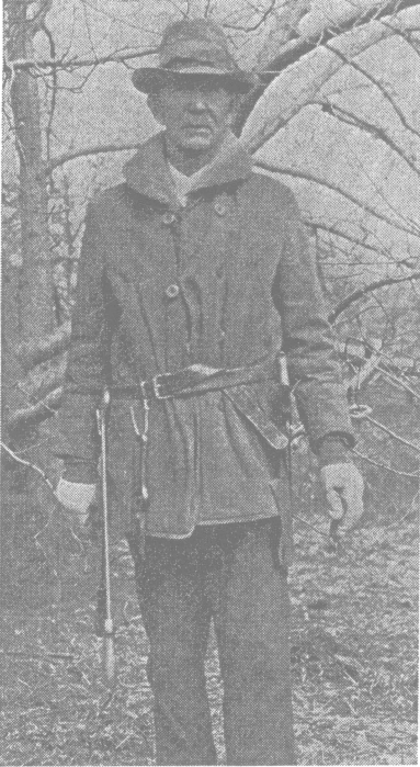
Fig. 2.—A heavy leather belt supplied with wire hooks on which to hang tools is very handy while working. Swivel bladed orchard pruning saw, hand shears, and lopping shears, are hanging from this belt.
