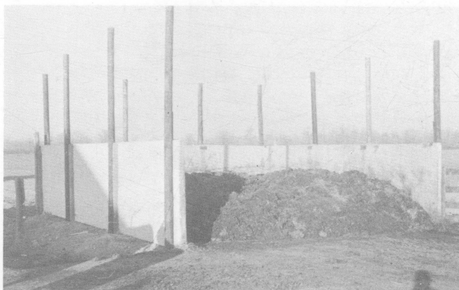
Some dairymen with free-stall housing use above-ground storage such as the above
