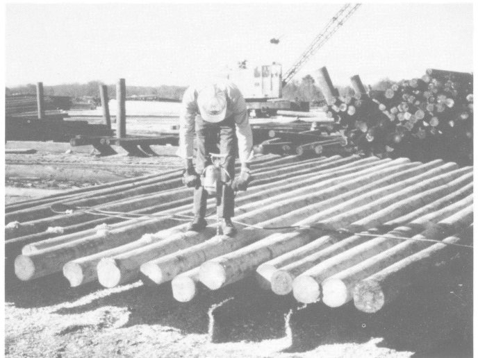
All sawing, drilling and other framing work should be done prior to treating the wood.
