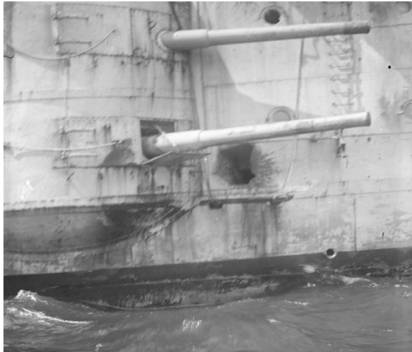
Figure 9: Vickers BL 6-inch Mark VII naval gun (seen here on HMS KENT)
