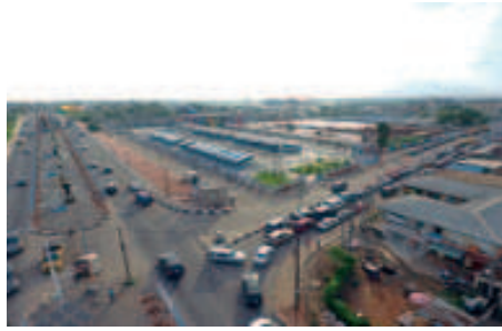
Ikeja Bus Terminal – Before & After
