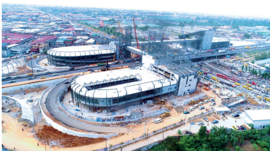
Aerial picture of the completed Oshodi Transport Interchange
