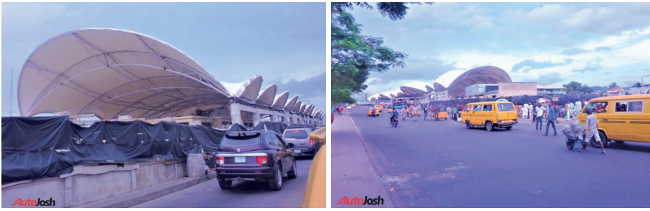
Yaba Bus Terminal (currently under construction)
