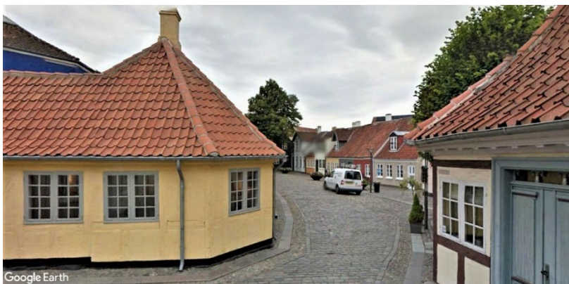
Figure 5. The yellow washed corner building is the humble dwelling where H. C. Andersen was born. When built it was more fashionable with regular brickwork than half-timbered constructions. Therefore, the timber is yellow washed like the rest of the wall in contrary to the building to the right where the timber frame is expressed. Google Earth 2019
