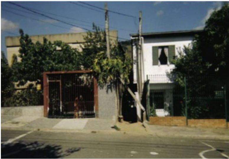
Figure 2 - High quality auto-constructed homes preserved in the participatory slum upgrading process, Vila Radiante, East District, Porto Alegre. Photo credit: Ana Paula Pimentel Walker (Walker, 2016).
