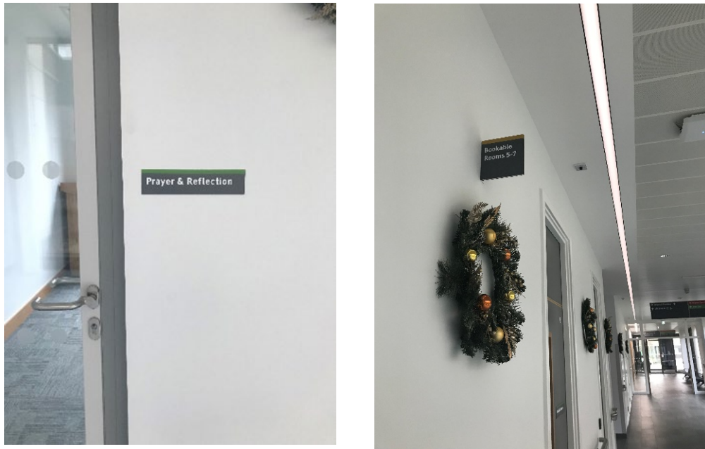
Figure 11 &12. Wall fixed and protruding wall fixed signage.
