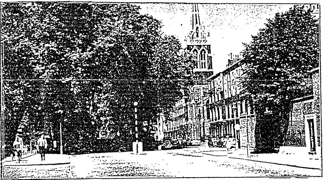
Fig. 2.16 Photo of Worburn Square before demolition (Photo by the author, C. Ward.)
