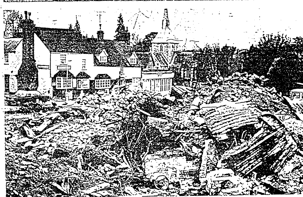
Wheathampstead, Old Town Farm, before and after demolition
