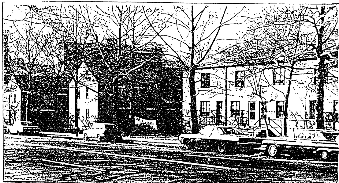
Fig. 3.1 View of Clason Point Gardens from bordering Street, before modifications (Photo by author Oscar Newman)
