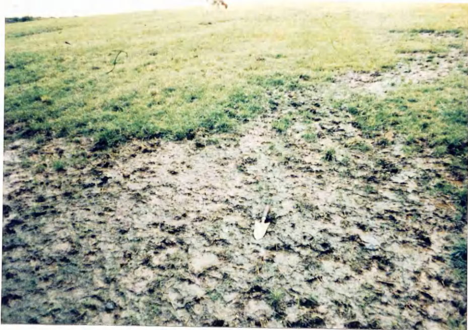
PLATE 9 - ENTERKINE - Damage to soil layer.
