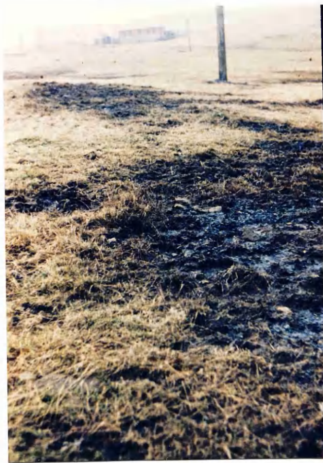
PLATE 14 - BANK - Damage to soil layer and vegetation cover due to pyrite oxidation in underlying spoil.
