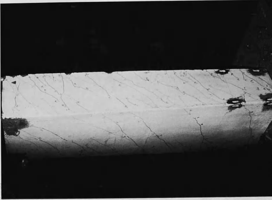
Plate 8.12 Crack pattern in the back wall and side wall 2
