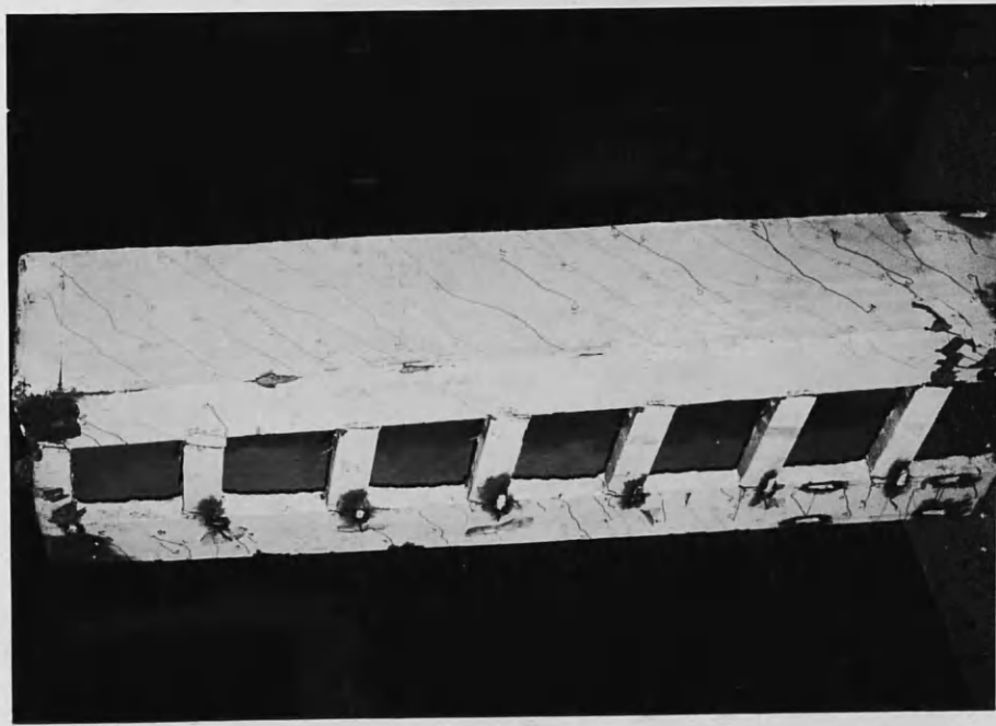
Plate 8.11 Crack pattern in the front wall and side wall 4 (Model 1)
