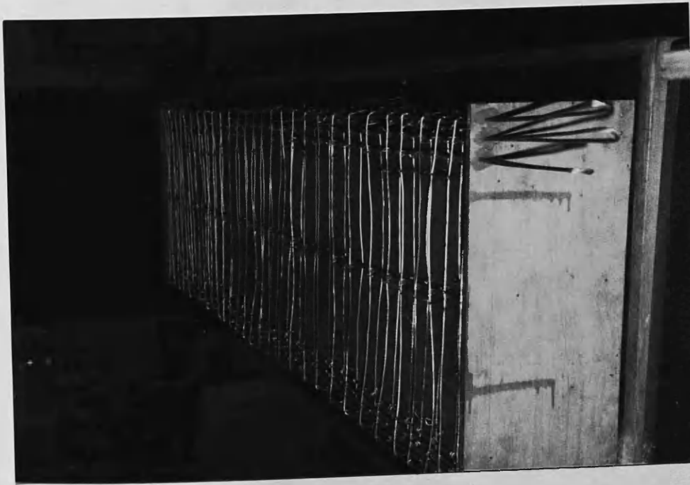
Plate 8.5 Inner shuttering and reinforcement of the back wall (singly symmetrical model)
