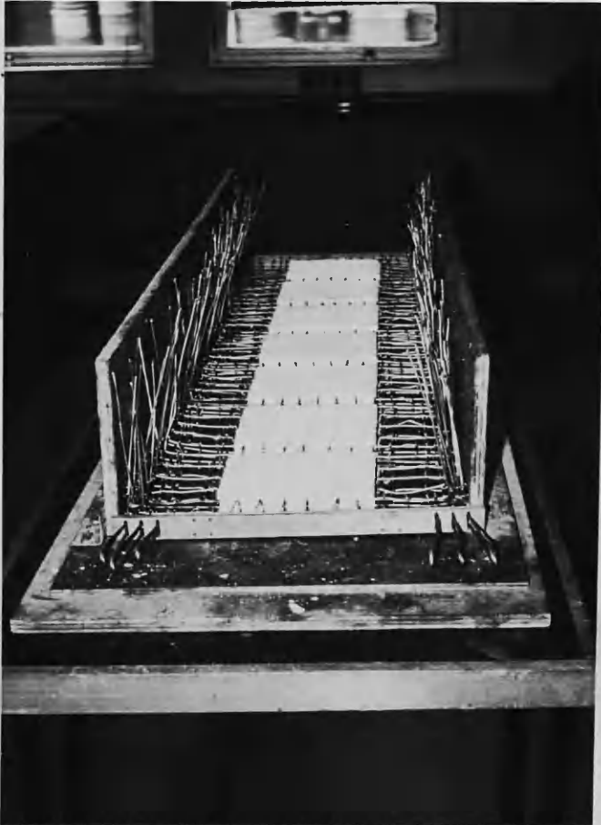
Plate 8.4 Outer shuttering and reinforcement of the front wall
