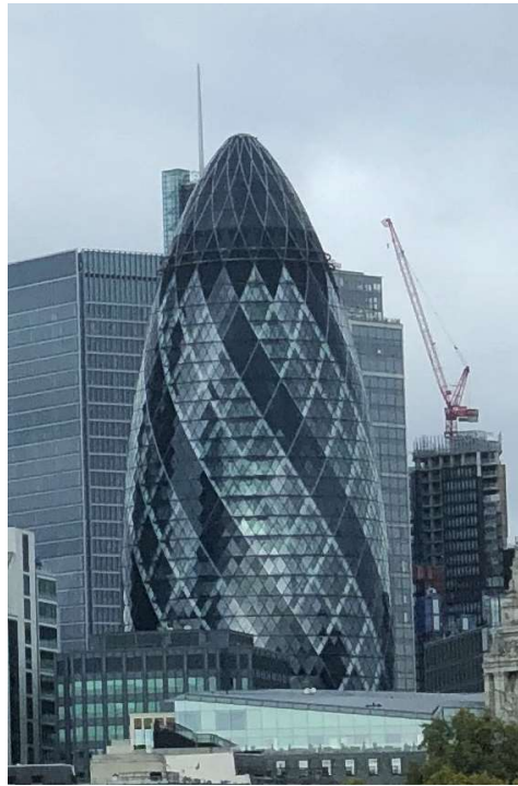
Fig 1: An example of Diagrid Tube Structure: Swiss Re Building, London
