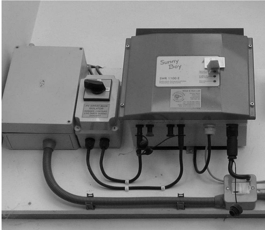
Figure 7. Poor provision of energy feedback in the installed inverter in case study C
