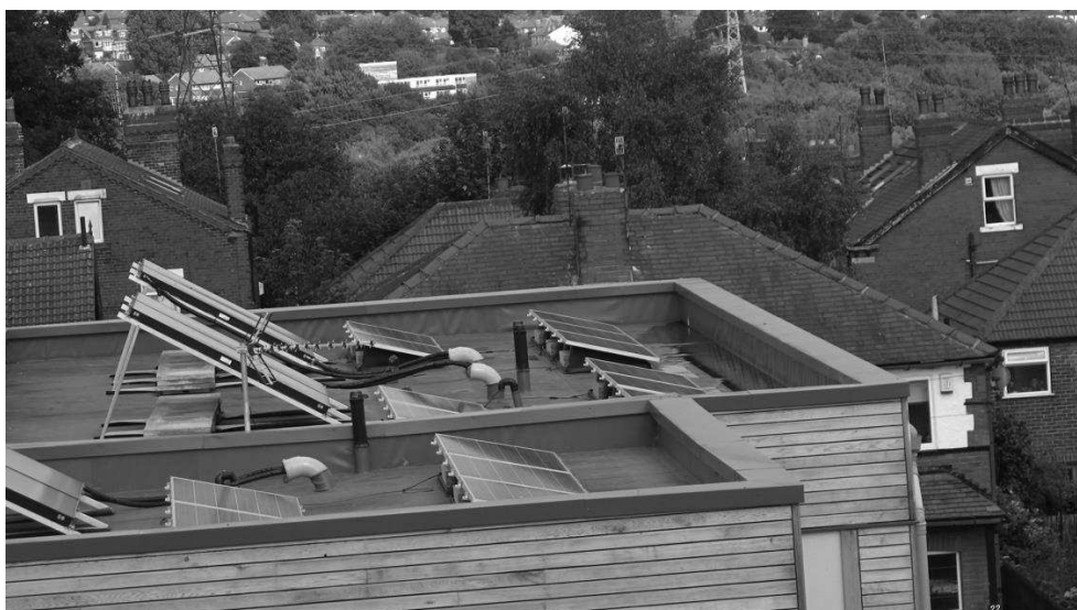
Figure 9. Inaccessible and hidden PV panels (A)
