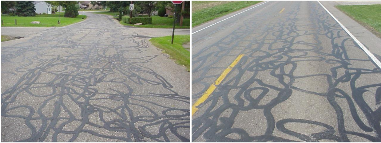
Figure 2. Extensive Crack Sealing in Flexible Pavements
