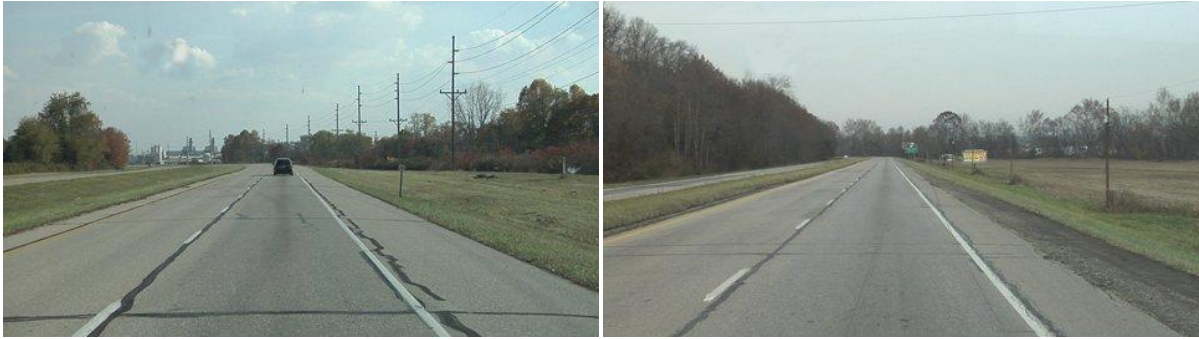
Figure 4. Sealing Reflection Cracks in Composite Pavements
