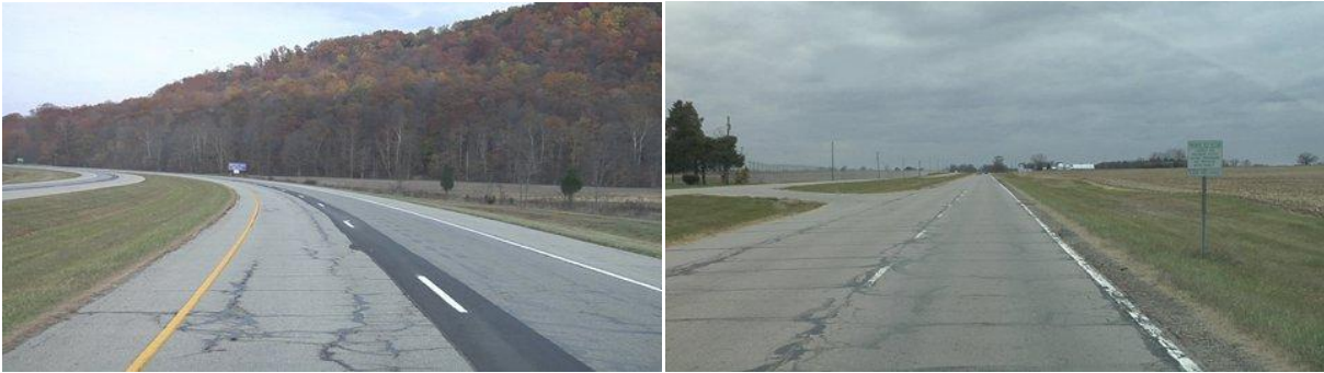
Figure 3. Sealing High Severity Cracks
