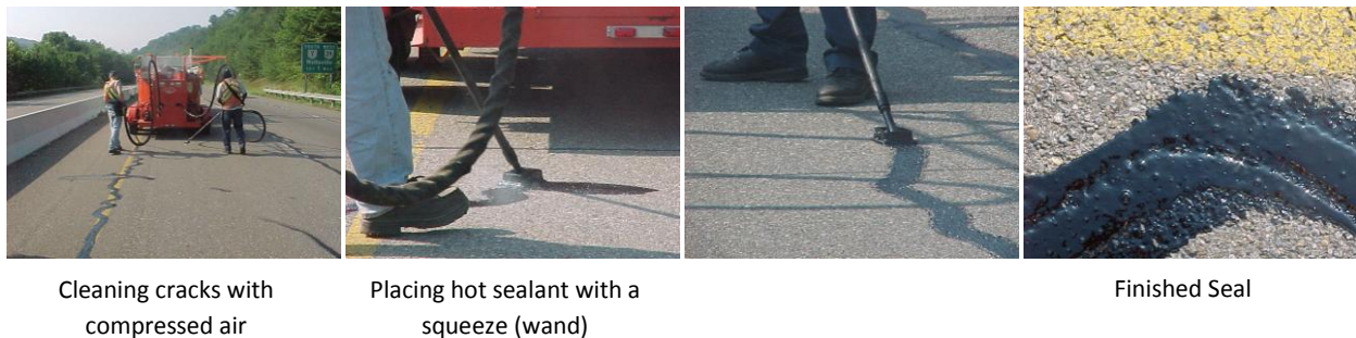
Figure 1. Crack Sealing Operation
