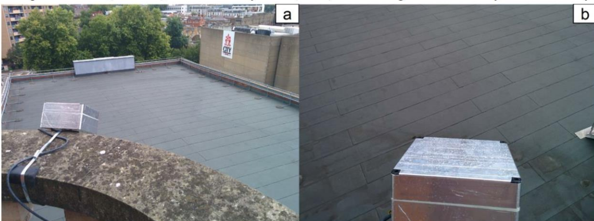
Figure S-5. Enclosed longwave infrared camera (camera C7) installed at the CUB site for atmospheric correction evaluation with its “short” roof-camera path length (a) mounted on a bell tower to the southwest of the target roof. Images 7 September 2017.
