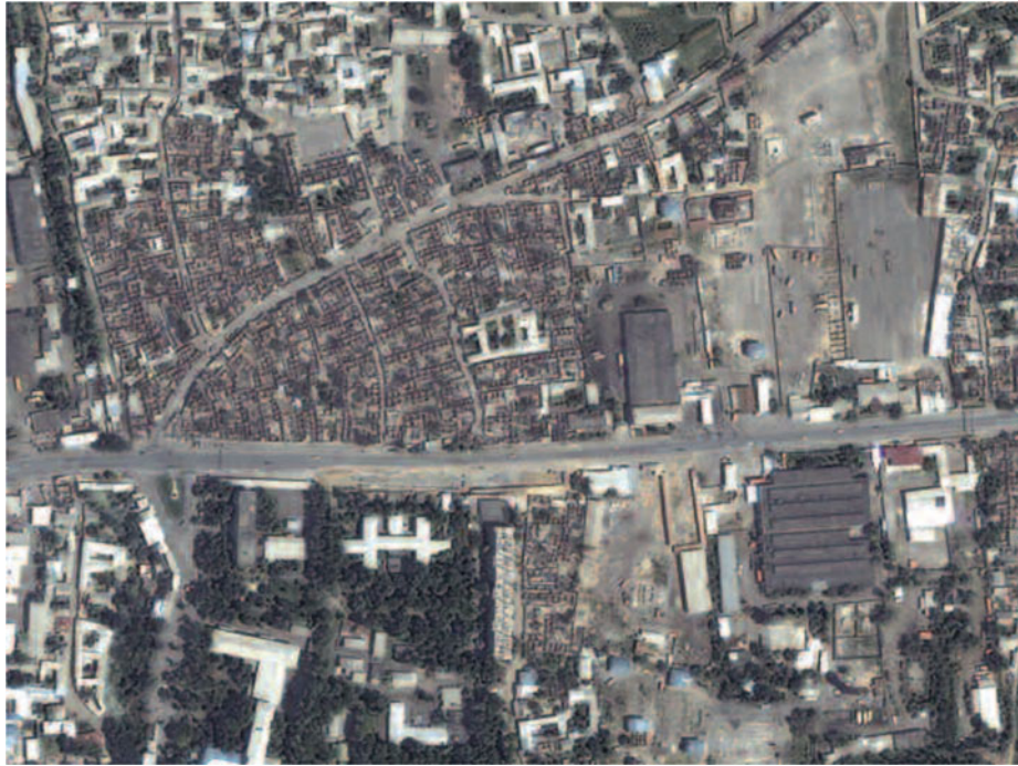
FIGURE 3. Destruction During the 2010 Osh Riot (Detail)
