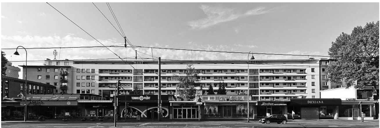
Figure 19. W. Riphahn, Hahnenstrasse complex (1945–1952). Source: Spekking (2014).
