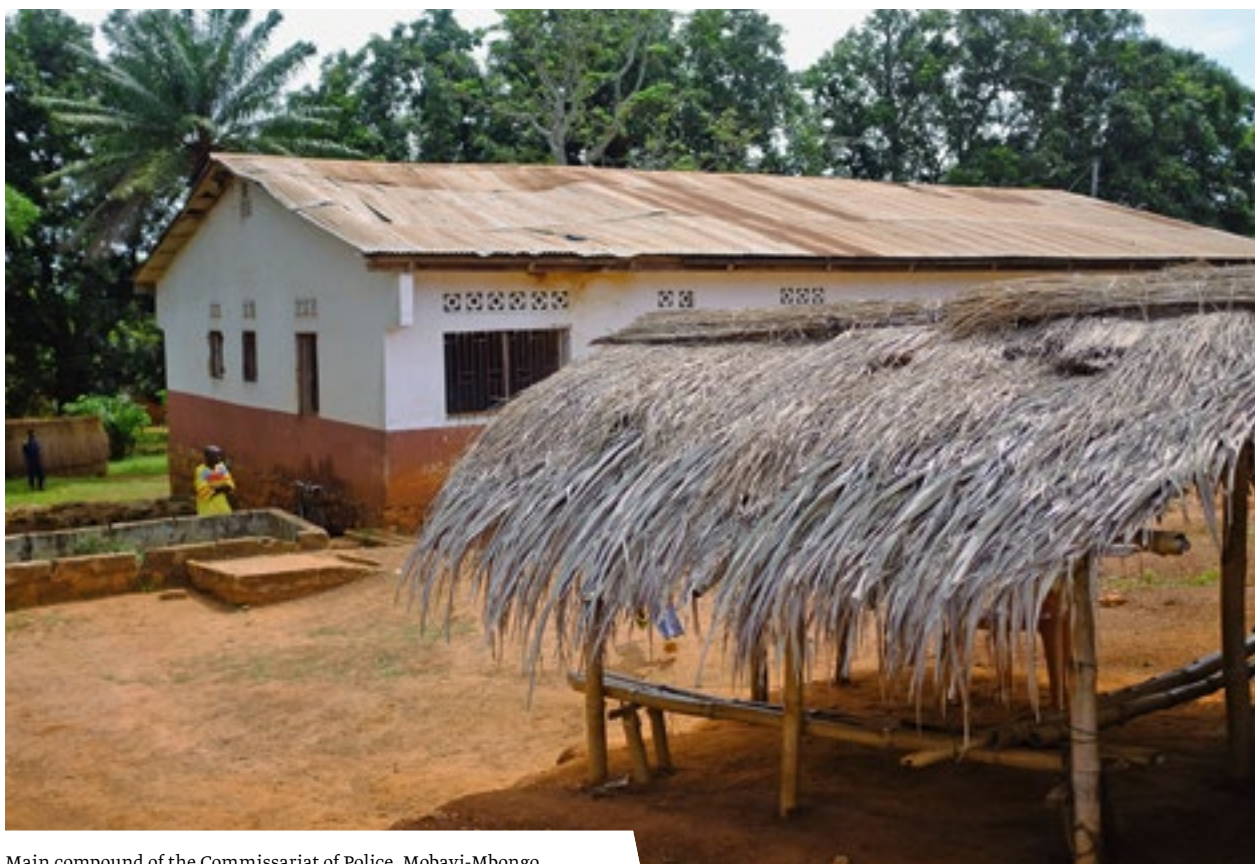
Main compound of the Commissariat of Police, Mobayi-Mbongo
