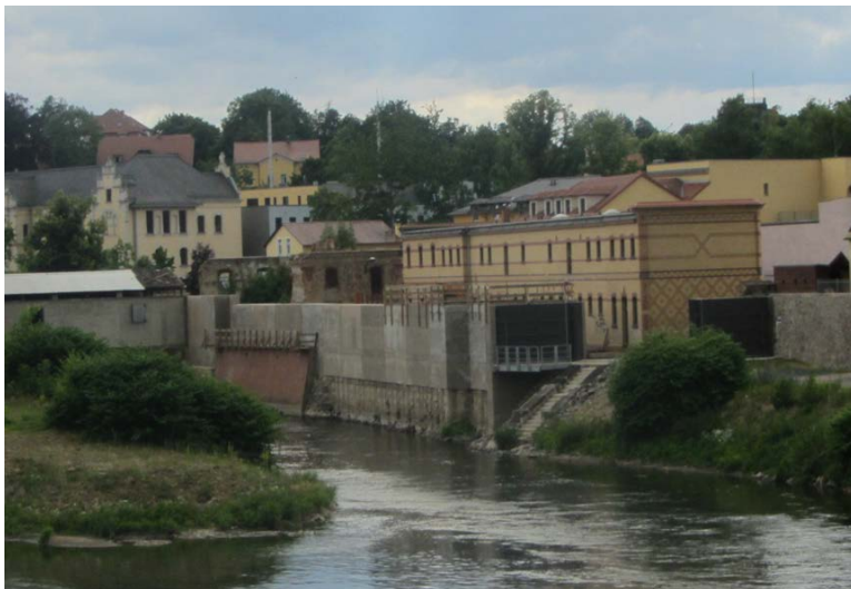
Figure 4 Floodwall, Project 2, under construction (June 2017, authors).
