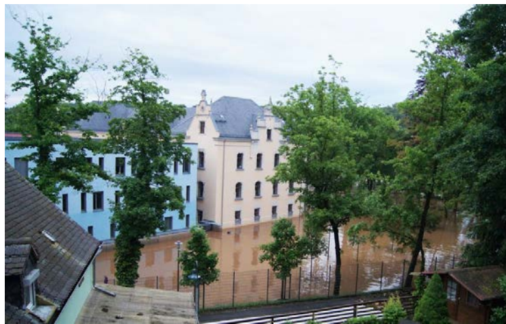
Figure 34 New police station flooded during the 2013 flood (Colditzer-tageblatt online newspaper, 2013)
