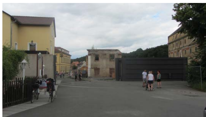
Figure 27 Floodgate, part of the floodwall Project 1
