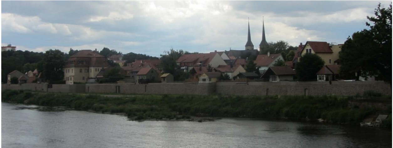
Figure 33 New floodwall, photo taken across the Mulde River by the authors (June 2017)
