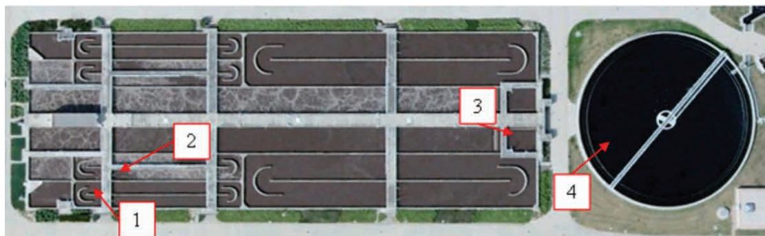
Figure 1. Sampling sites within the Central Wastewater Treatment Plant in Koziegłowy: 1 – bioreactor tank 1; 2 – bioreactor tank 2; 3 – bioreactor tank 3; 4 – secondary clarifier.
