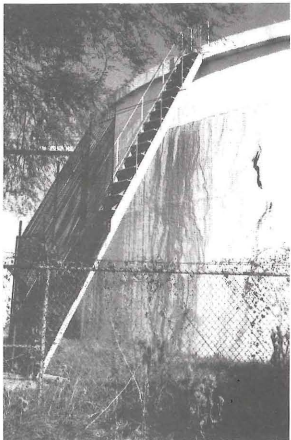
Figure 16. View north-northwest of the west side of the eastern Bedell tank, 1997.
