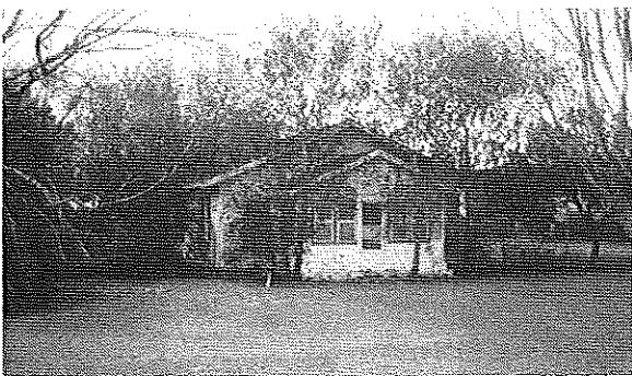
Figure 25. Looking south-southwest at the J. A. Weslander House.
