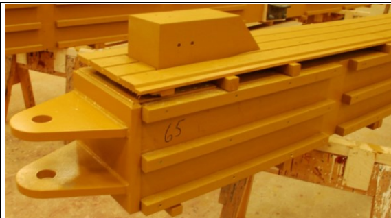
Fig. 7. Weather protection of the arch. Ventiladed wood panels are attached to the sides of the arch, whereas a coated steel sheet is applied on the top (not applied yet at the time when the picture was taken).
