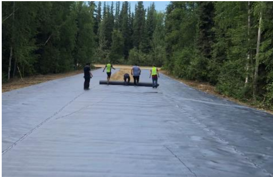
Figure 3.22 Installation of the wicking fabric
