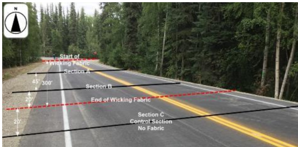
Figure 3.18 Test section layout at Toklat Way
