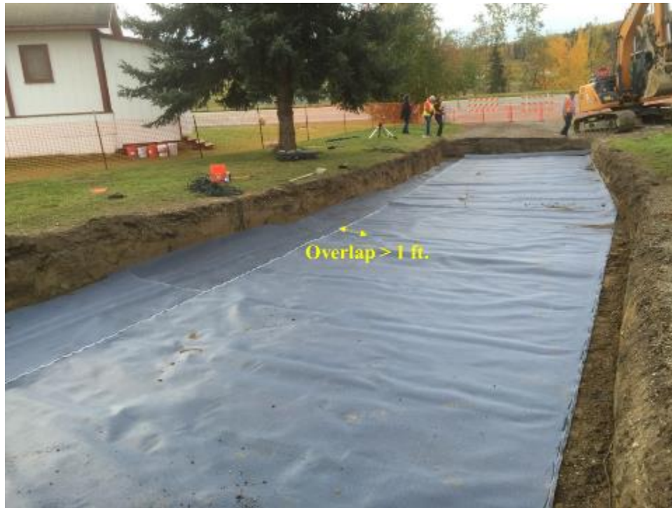
Figure 3.9 Installation of H2Ri wicking fabric
