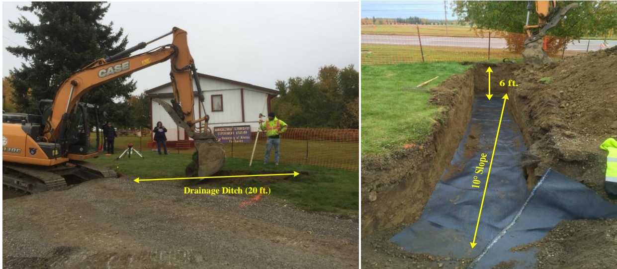
Figure 3.10 Excavation of drainage ditch
