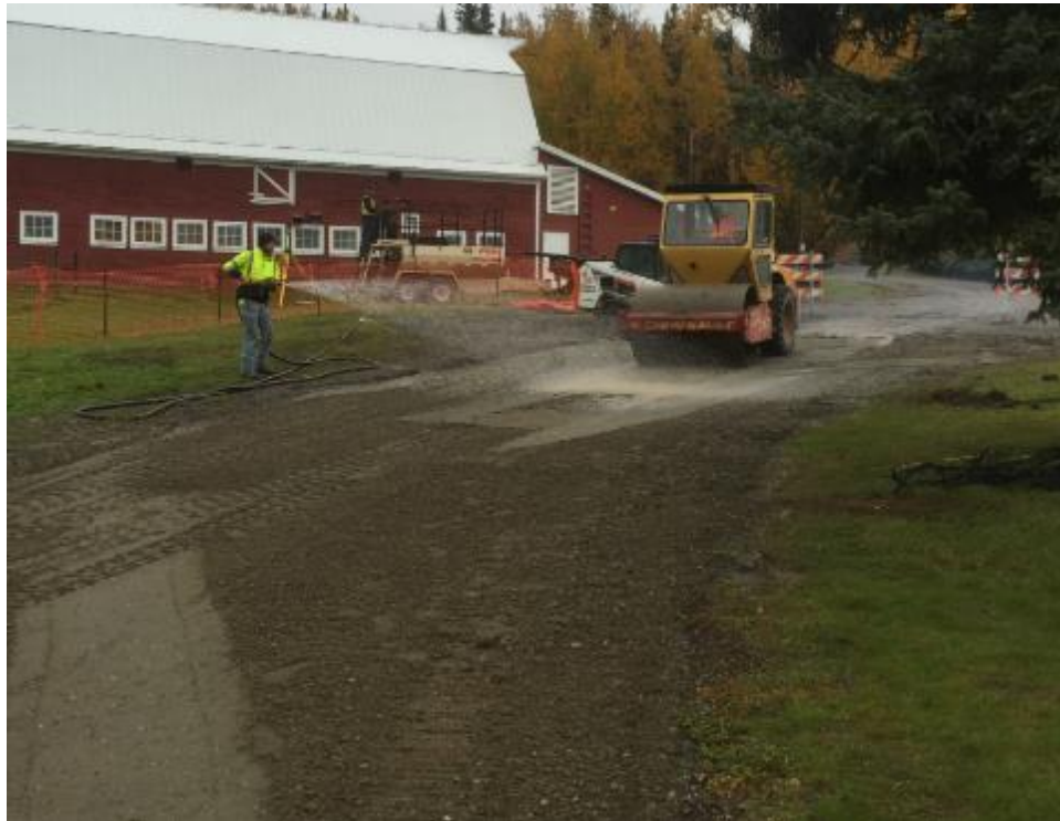
Figure 3.12 Compaction of Type A fill
