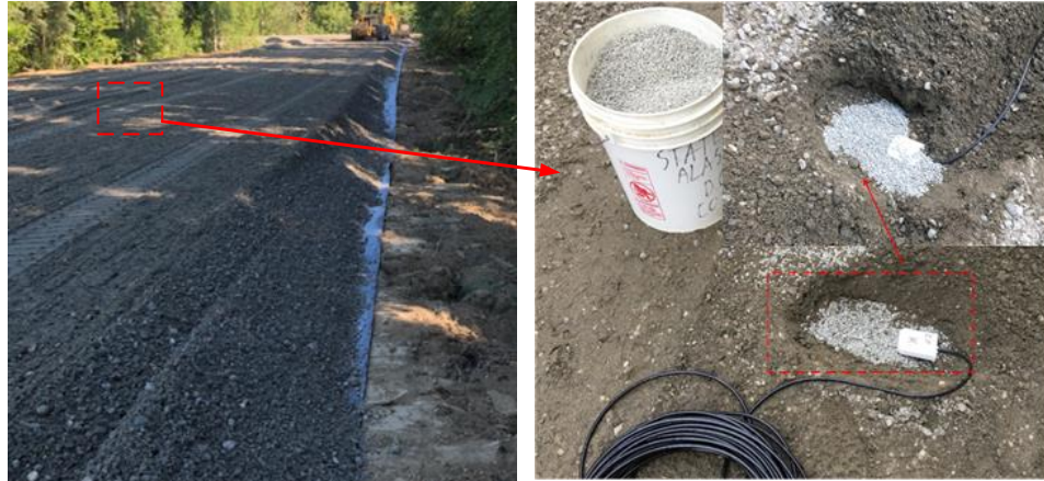
Figure 3.23 Installation of the 2 nd layer of sensors
