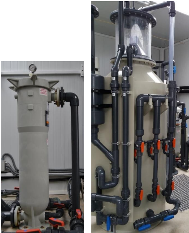
Figure 10: Water filtration system used at Riasearch. At the left: suspended solids filtration system; At the right: protein skimmer, to remove dissolved solids. Photographs by Ariana Laranjeira, Riasearch.
