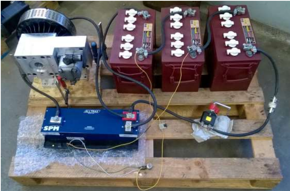
Figure 5.59 – Assembly for the first electrical test, May 2015
