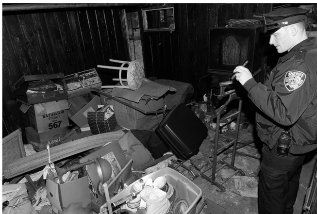
Figure 3: Damage Inside Merin's Home 20
