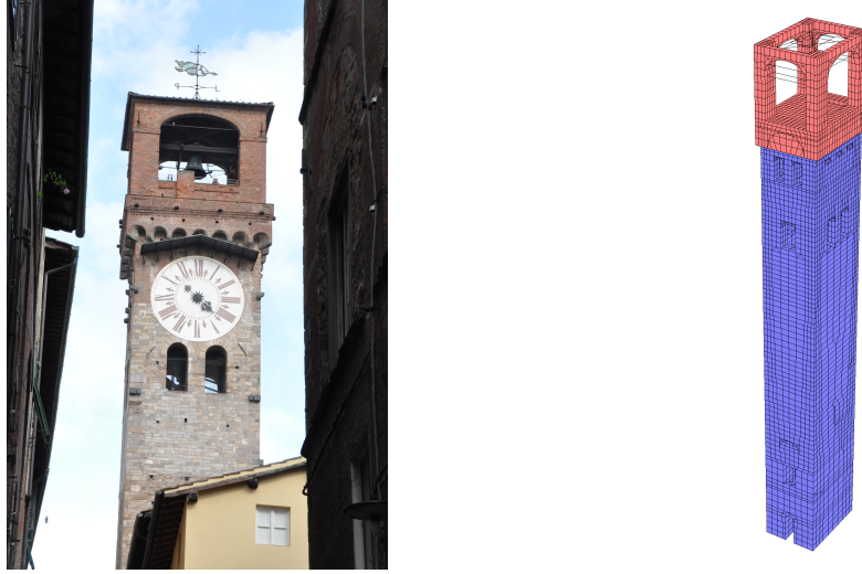
Figure 10: On the left, a picture of the clock tower in Lucca. On the right, the mesh used for the finite element discretization, where the different materials for the bell chamber and the lower part of the tower are reported in different colors (respectively red and light blue).
