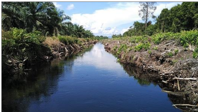
Figure 2.7 The ditch at the border of DF with a width of 3 m, and about 1.2 km away from tower.
