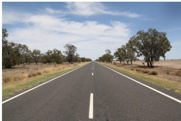
Figure 4: The dry and parched land throughout rural areas in Australia
