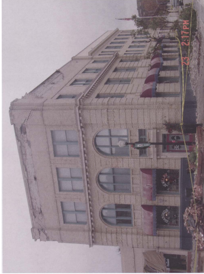
▲ Figure 14. Upper left: Collapsed Acorn building on the corner of 12th and Park Streets in downtown Paso Robles (photo by Rakesh Goel). Upper right: Bistrot Laurent building with seismic retrofit survived the earthquake; inset shows bolts from retrofit (photo by Rakesh Goel and Khalid M. Mosalam). Lower left: Facade damage of Ali's Persian Rug building at the corner of Park and 13th Streets (photo by Khalid M. Mosalam). Lower right: Collapsed wine barrel stacks at Turley Wine Cellars, Highway 46 West, Paso Robles (photo by Josh Marrow).
