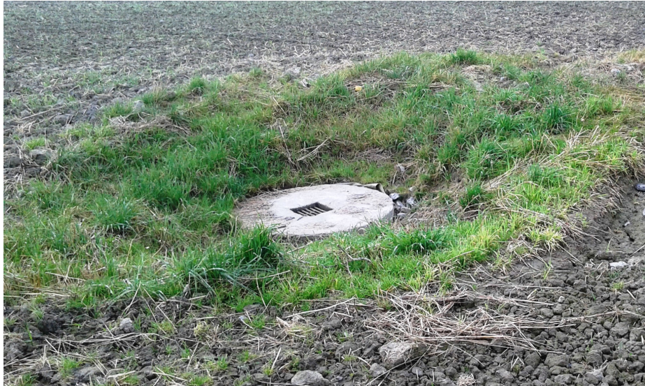
Figure 13. Restored manholes in Mørdre (photo: Stine Vandsemb)
