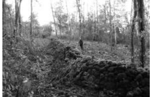
Fig. 10 - Section of self-standing dry stone wall made visible by forest harvesting activities.
