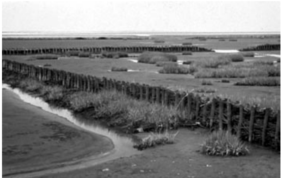
Fig 11. Soft structures for sediment control along the North Sea
