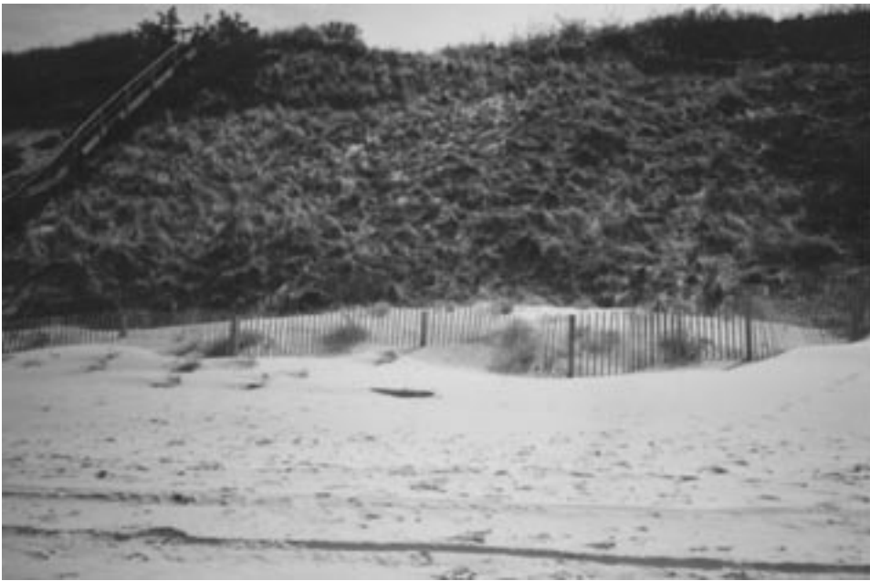
Fig 29. Completed bank stabilization project
