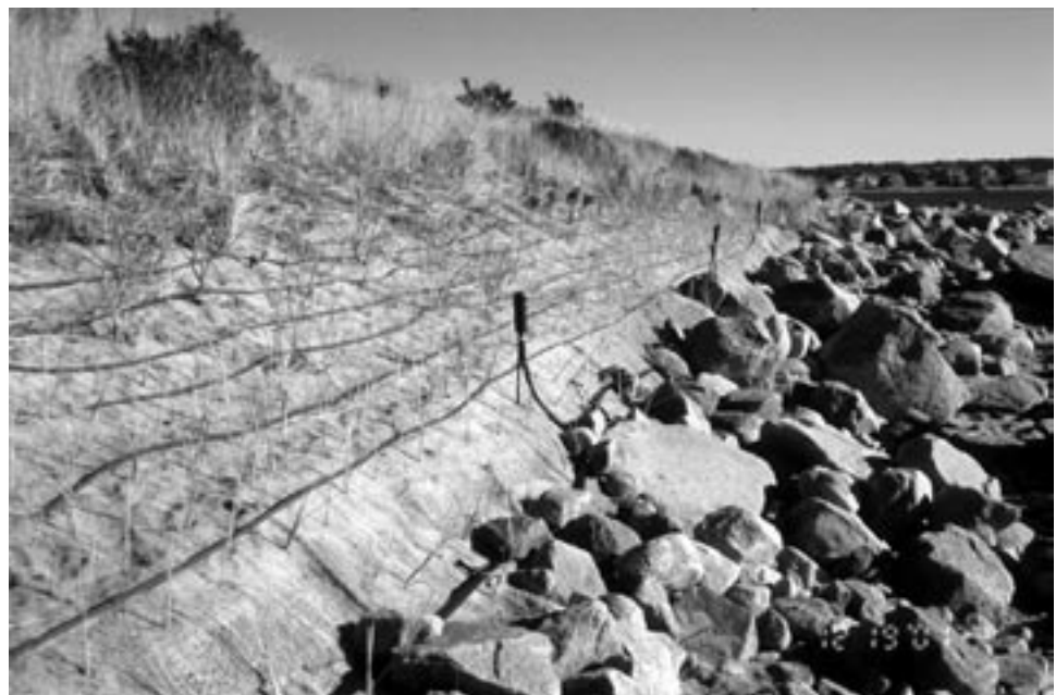
Fig 7. Coastal bank erosion control using bioengineering (bio-logs, jute netting, plants) and a system for watering and fertilizing
