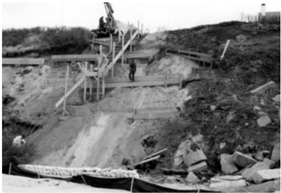
Fig 27. Terraces built across the coastal bank
