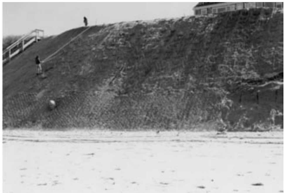
The next step was Fig 28. Coastal bank with fill and jute netting being planted
