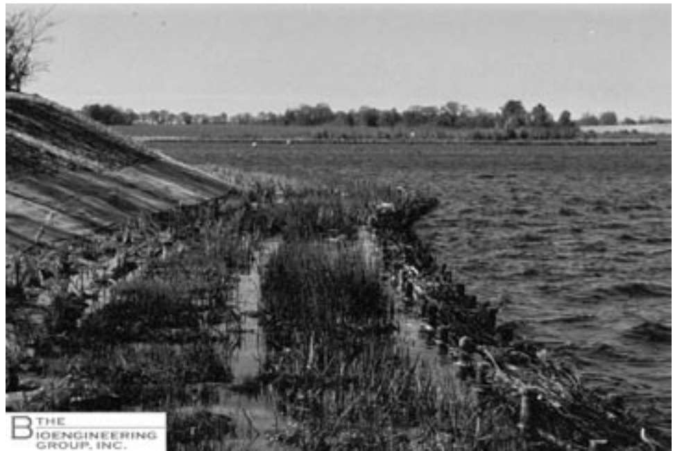
Fig 12. Sediment control using soft breakwaters & sills
