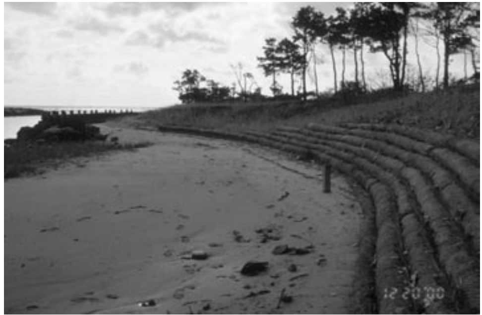
Fig. 8: Well designed bioengineering for coastal bank erosion control
