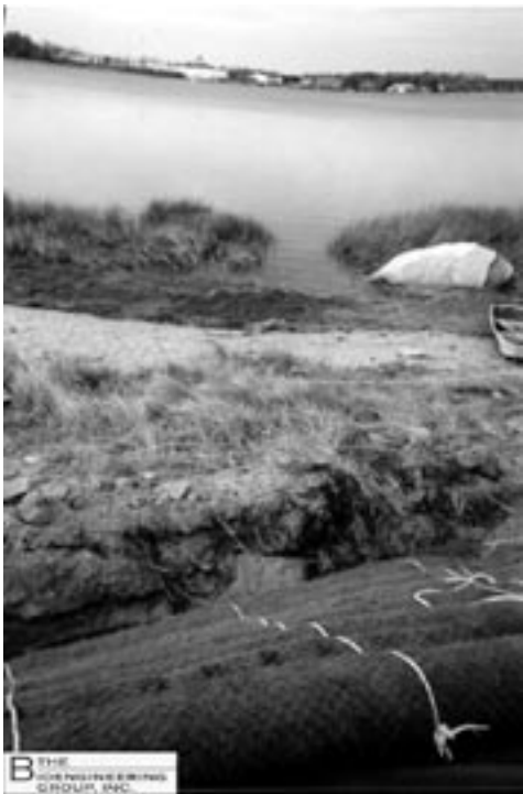
Fig 14. Coir fascine for bank stabilization
