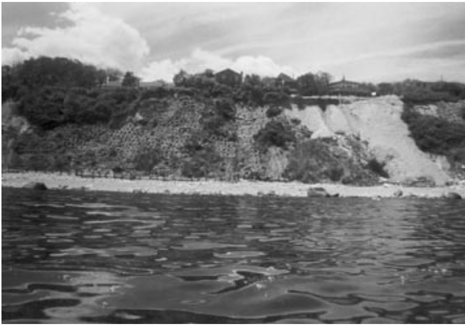
Fig 1. Innovative non-structural erosion control methodology on a coastal bank: A matrix of hay bales
