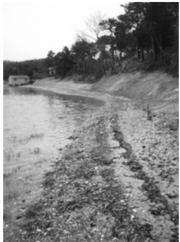
Fig 34. Bournes Pond bank stabilization project completed
