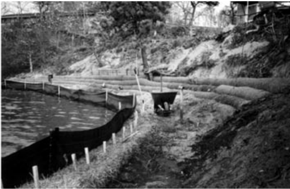
Fig 33. Bournes Pond bank stabilization under construction
