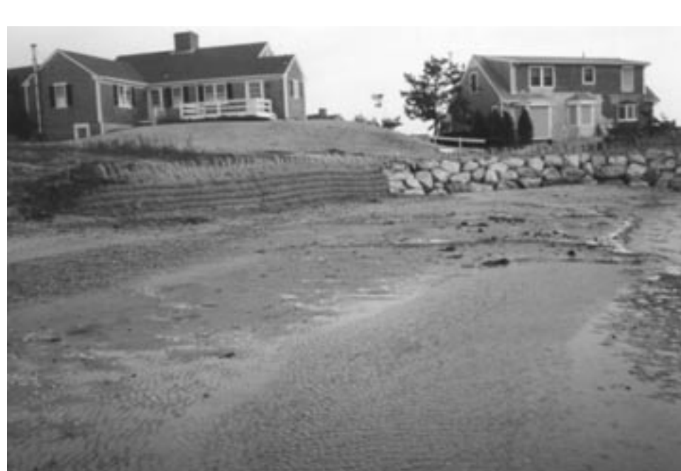
Fig 36. Using fiber rolls to construct a return
